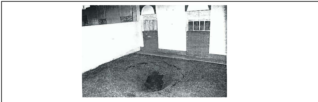
Figure 8. Cesspool collapse and sinking in a backyard in Pizarro neighborhood, Río Cuarto city as a result of the rising watertable in 1999 (Photograph from “Puntal” newspaper).
