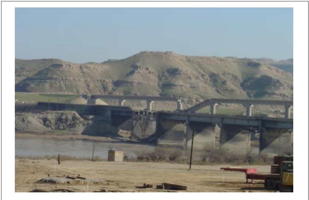
Figure 1. Al Fathah Bridge from west side.
