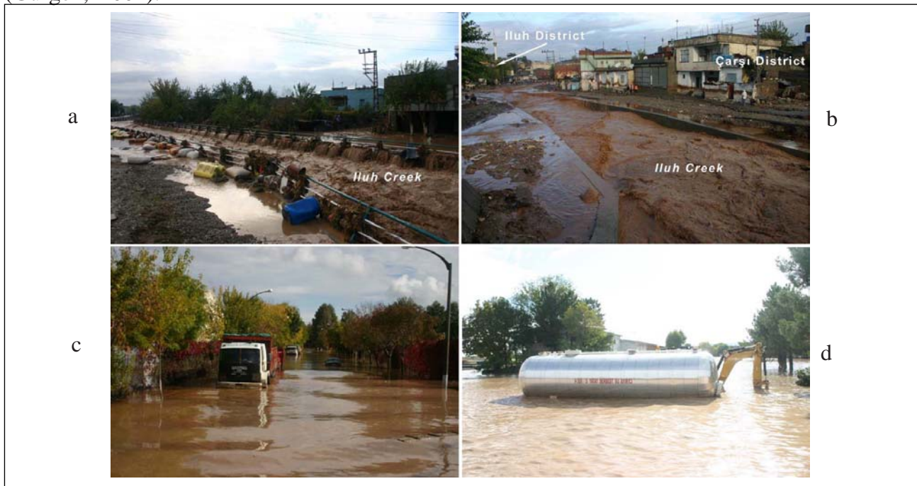
Figure 2. Treatment channel built on the part of Iluh Creek in the city center of Batman (a,b - dwellings built on the former stream bed around the channel were considerably affected by the flood in 2006. c,d - great torrents occurred around the channel after the flood).
