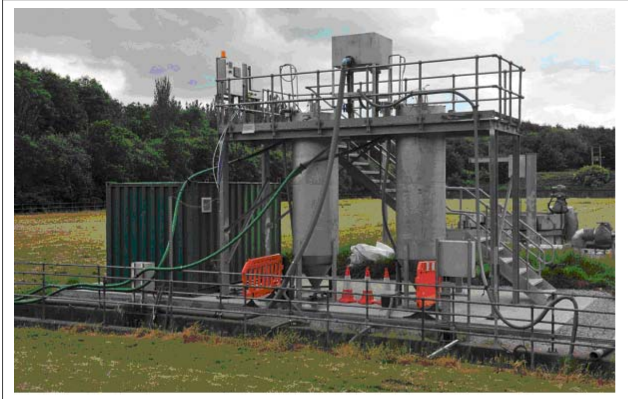
Figure 2: The pilot plant on site showing the two filter units with the common header to equalise flow..
